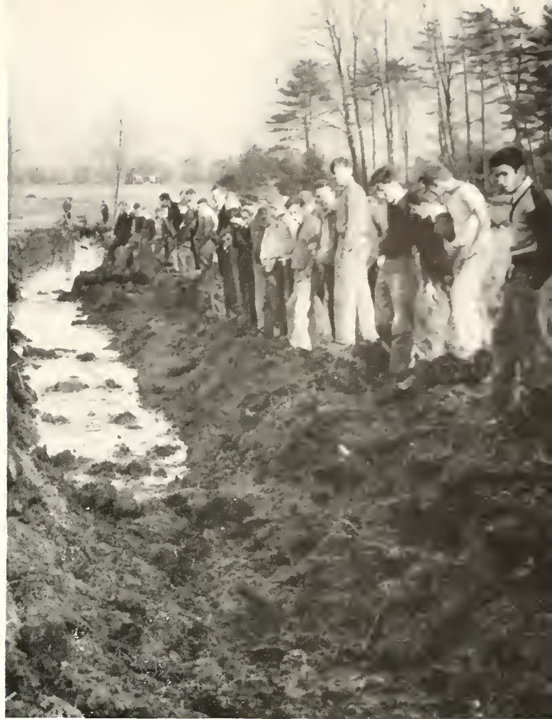
This is how the ditch looked when the class returned to inspect the results of the blasting. Students study and apply on their farms practical methods in farm mechanics.
